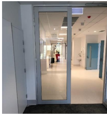
Luminance contrast is not achieved due to floor finish colour.
